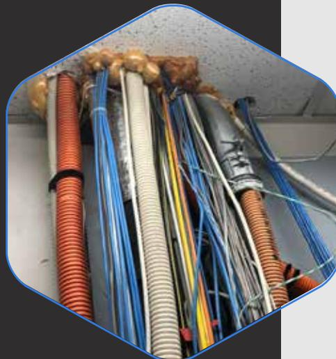
Unmanaged riser closets eventually become aesthetically unappealing and reach conduit or core hole capacity (pathway congestion), impacting the ability to provide reliable service to your building and tenant networks and costing ownership time and money to remediate.
